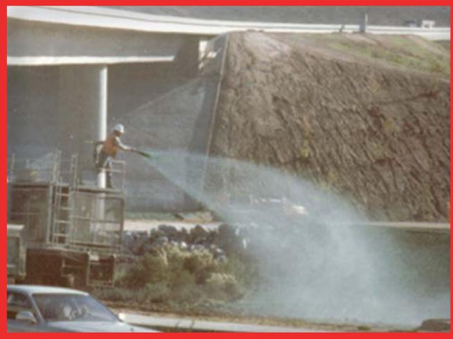
AM 120 Mycorrhizal Inoculant applied through hydroseeding equipment.
